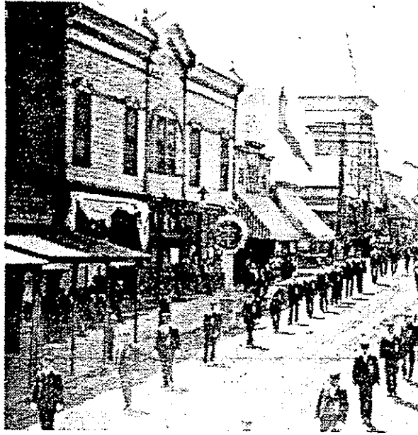
HISTORICALLY, ALL STOREFRONTS ALIGNED WITH CANOPIES AND AWNINGS AT THE SIDEWALK
